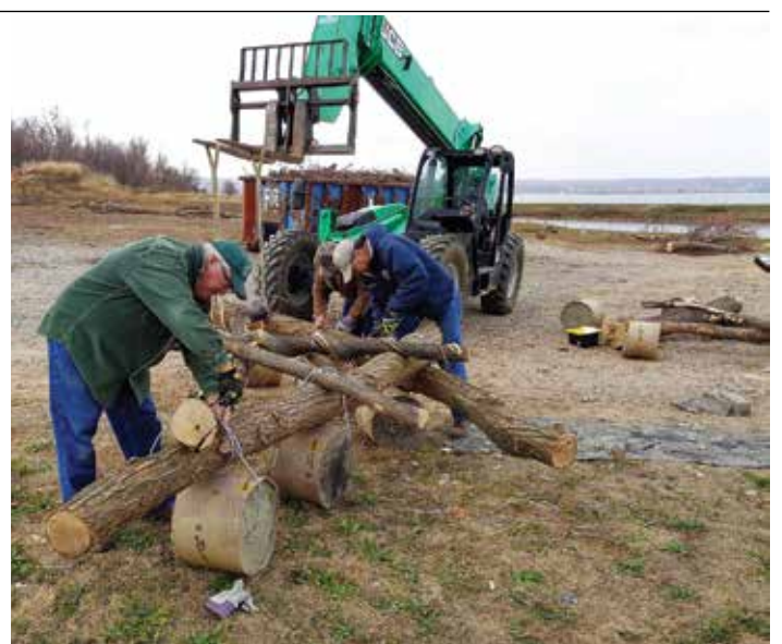
Scott and crew working on fish habitat structure.
